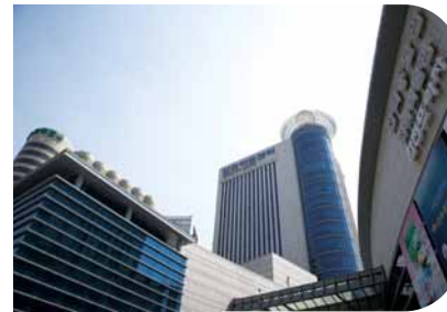
KEPCO Art Center, a cultural multiplex with a multi-purpose auditorium, galleries and an electricity museum
