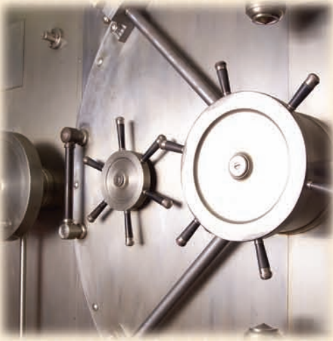
The vault pictured is located in our historic Charleston Broad Street office. Built in 1929, it is our understanding that the door alone weighs nearly six tons, and due to its massive structure, the vault was installed first and the building was built around it.
