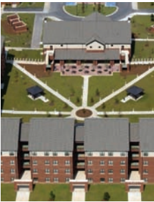
Fort Bragg 1st Brigade Barracks
