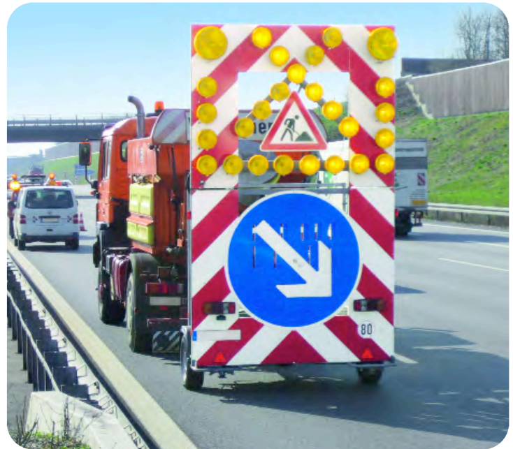
Traffic guidance system of Autobahnmeisterei München-Nord.
