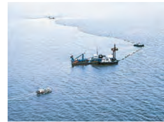
Dredging the mouth of the Barito River.
