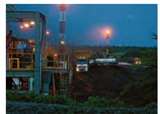
Dumping coal for crushing at the Kelanis River facility in the evening.
