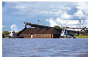
12. Barge loading at Kelanis
