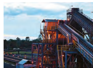
The Kelanis River Facility recently added an additional crusher to expand capacity to around 55Mt.
