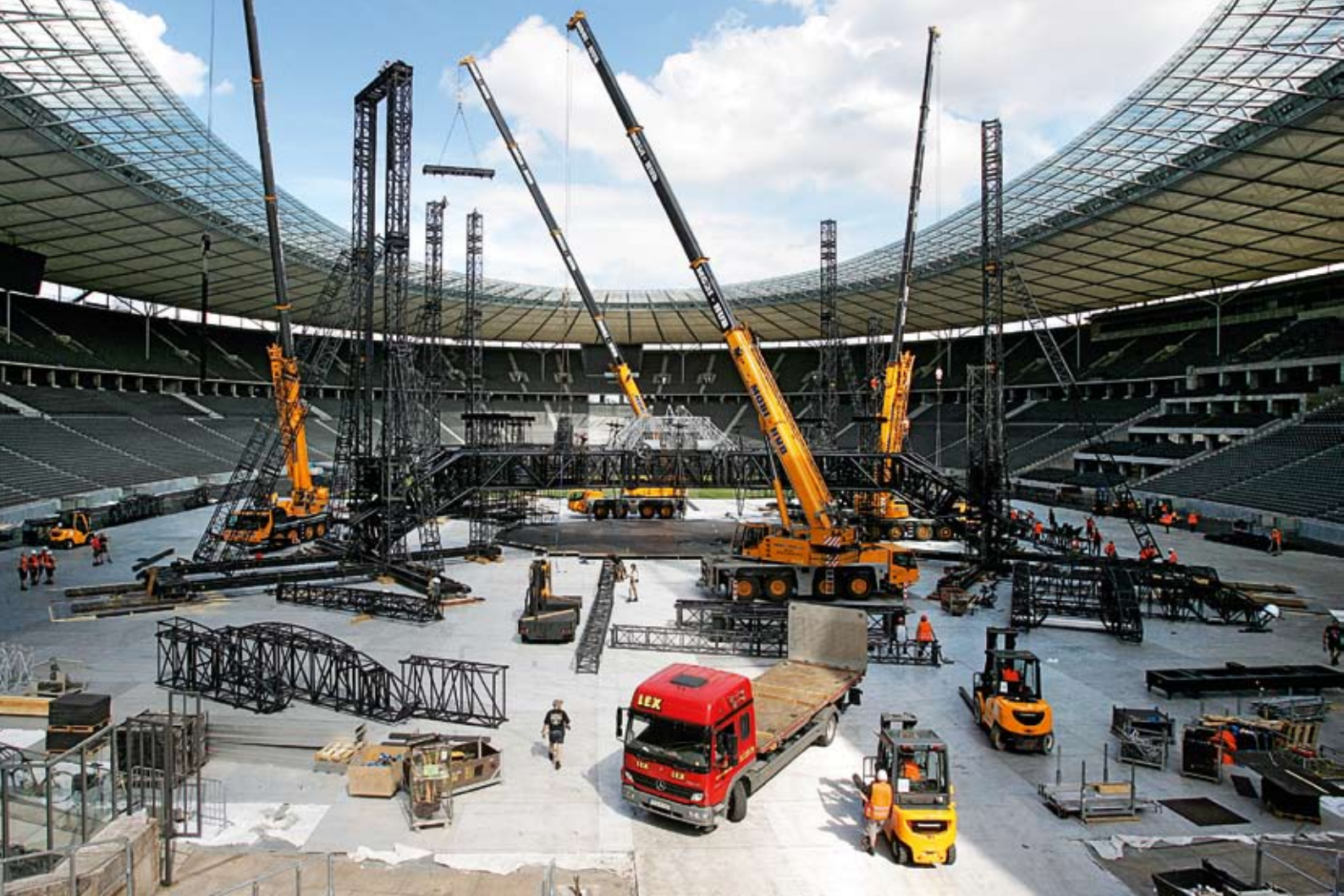
Dancing cranes: Builders need four cranes to erect the stage in the middle of Berlin's Olympic Stadium.
