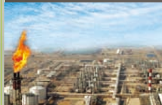
South Pars Gas Field Development Phases 4&5 Onshore Facilities, Iran (Mar. 2002 ~ Feb. 2005)
