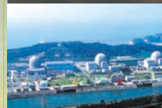
Yonggwang Nuclear Power Plant, Korea (June 1981 ~ Dec. 2002)
