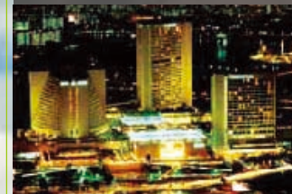
Marina Square Hotels & Retail Complex, Singapore (Mar. 1982 ~ Mar. 1987)
