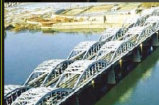
Han River Pedestrian Bridge, Korea (Sep. 1957 ~ May 1958)
