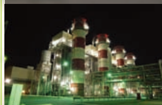
Zawia Combinde Cycle Power Plant, Libya (Feb. 2005 ~ Feb. 2009)
