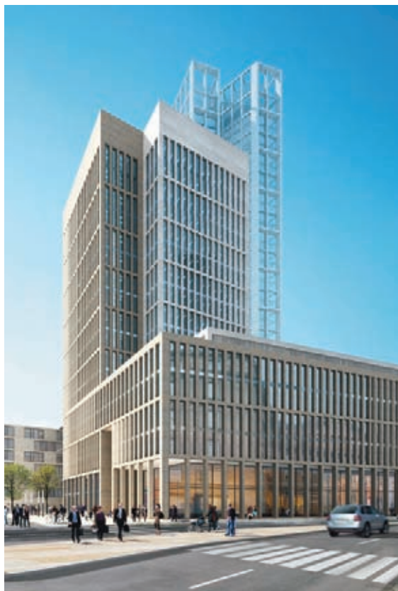
Frankfurt, Project MainTor
