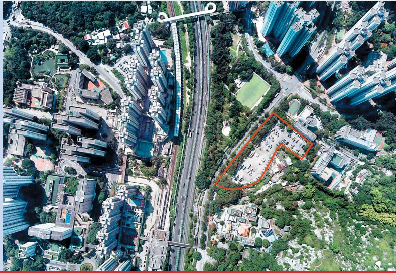
Aerial view of the site of Pak Wo Road project in Fanling 粉嶺百和路項目現址的鳥瞰圖
