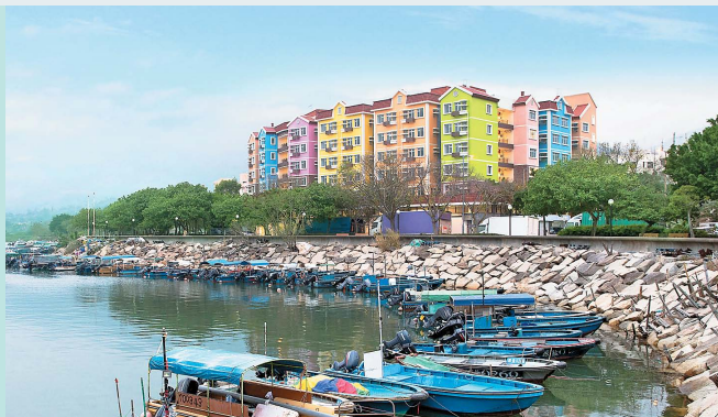
The design of Ying Hoi House is based on a European style village while maintaining the character of a local fishing community 迎海樓的設計富歐陸鄉鎮特色，亦不失本土漁村風味
