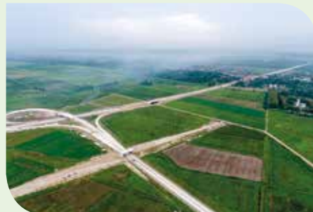
MEDAN-BINJAI TOLL ROAD - NORTH SUMATRA
