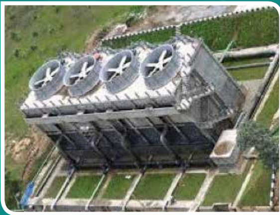
Cooling Tower is not a plural scene at the factory Cement, this WHRPG installation distinguishes Indarung -V factory with other factory.
