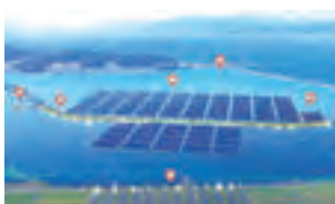
* Bird's-eye view of Floating Solar Power Site in Goheung Lake
