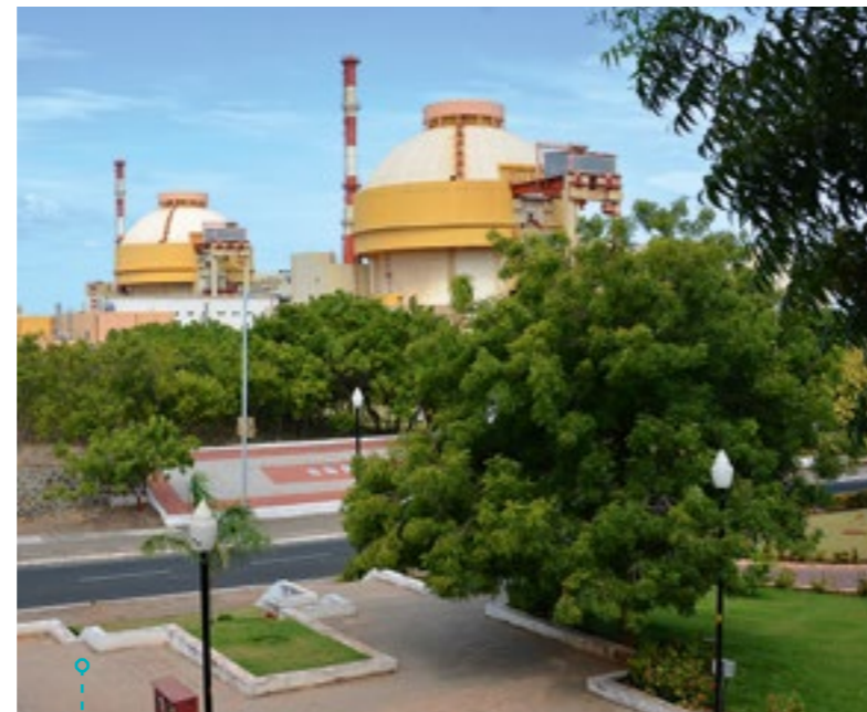
Kudankulam NPP (India) Units No. 1 & 2
