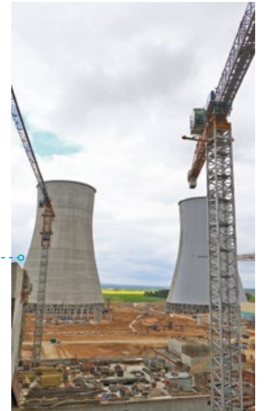
Belarus NPP construction, May, 2017
