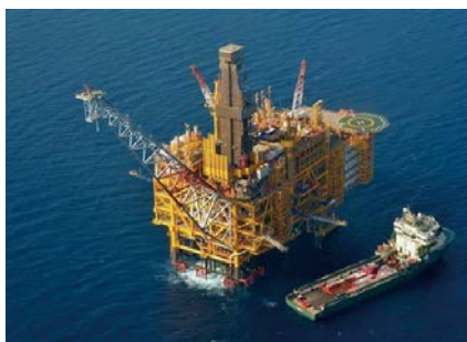
The Offshore Drilling Rig, Myanmar
