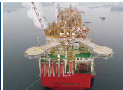
The FLNG Facilities in Prelude, Australia
