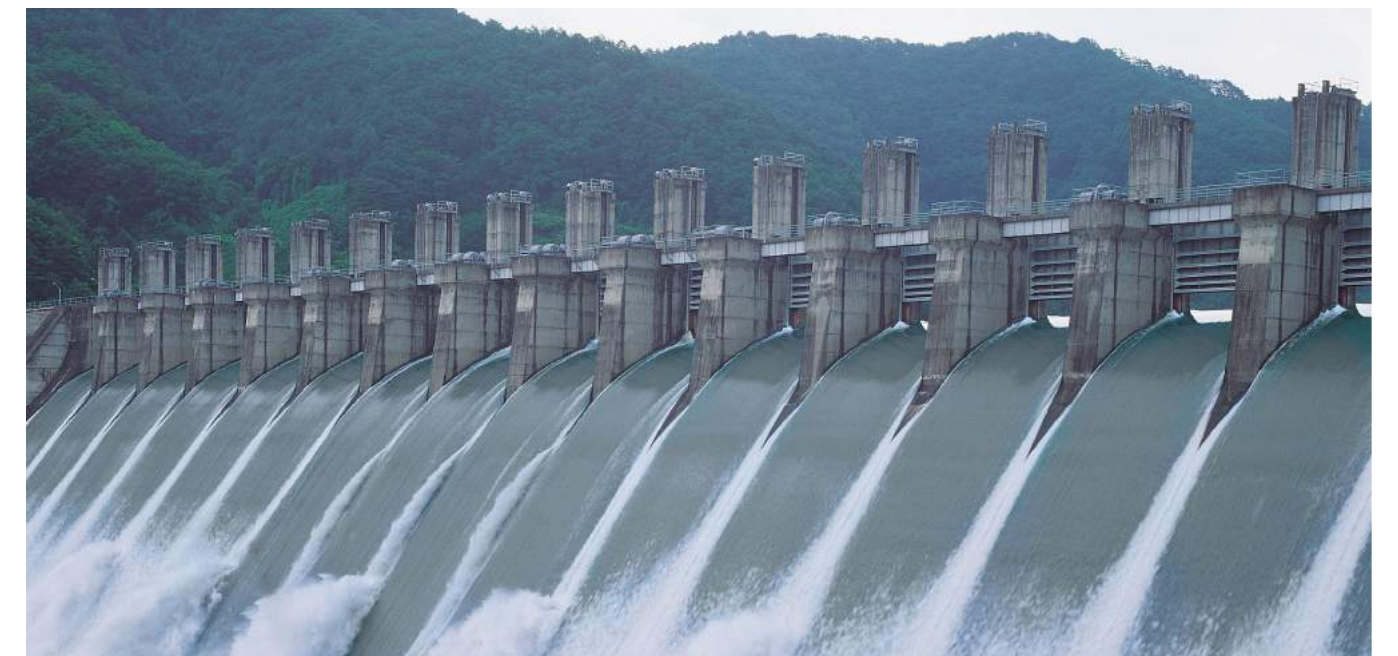
▲ Hwacheon Hydro Power Plant
