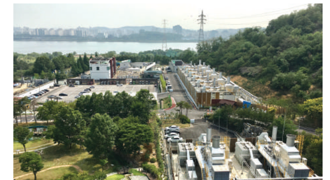
▲ Noeul Fuel Cell Power Generation Plant
