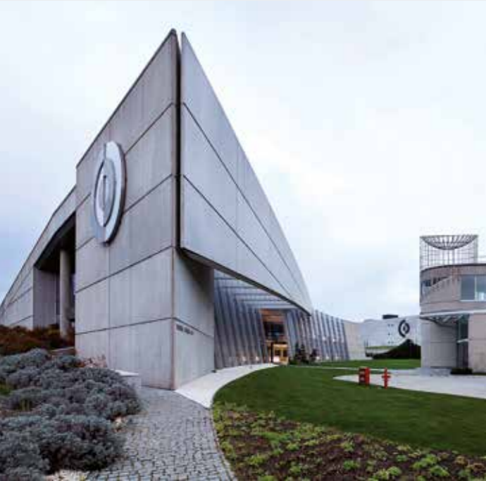
Abdi İbrahim Esenyurt Production Facilities
