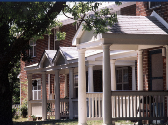
The Diggs Town community before scheduled renovations begin.
